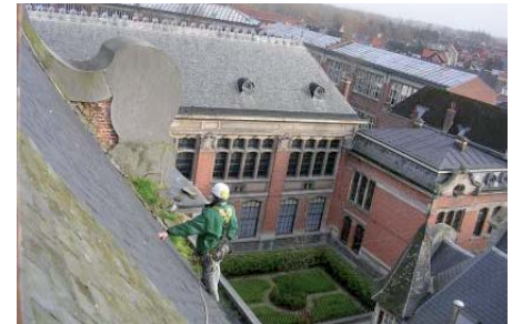
Assessing the roof of a heritage place using industrial rope access techniques
